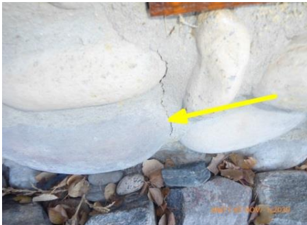
Fill cracks in rock veneer
