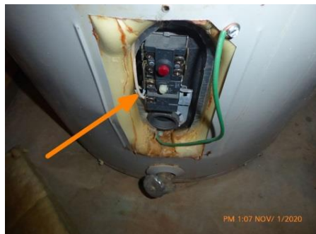
High Voltage Access Panel Removed by Others
